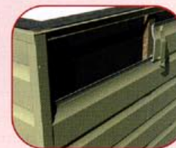
fig 10 Showing moisture barrier and battens before the cladding begins
