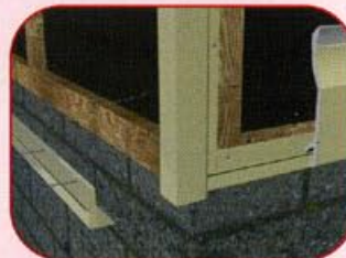
fig 8 Showing starter trim and showing the use of the universal corner trim for external angles
